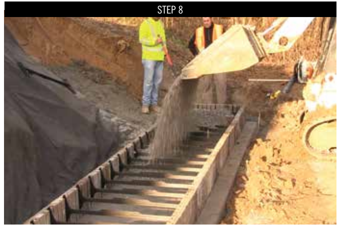
Place the #57 stone inside the Mega-Tandem™ (MSRW) panels to provide the internal gravel interlock. This will also provide for internal drainage to relieve hydrostatic pressure in the wall.
